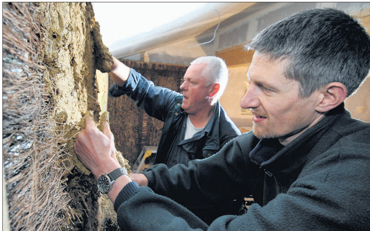
GETTING STUCK IN: Tom Mackeown, below left, shows Geoff Frost how to plaster with clay over straw bales
